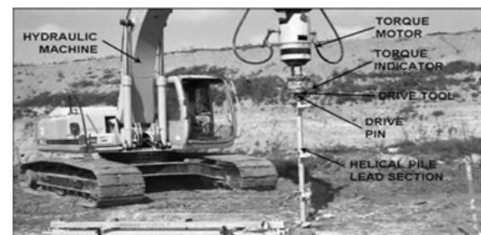
Figure 1: Installation of Helical piles with hydraulic machine
